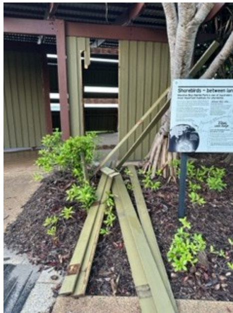
Vandalism at the Kakadu Beach Bird Hide
