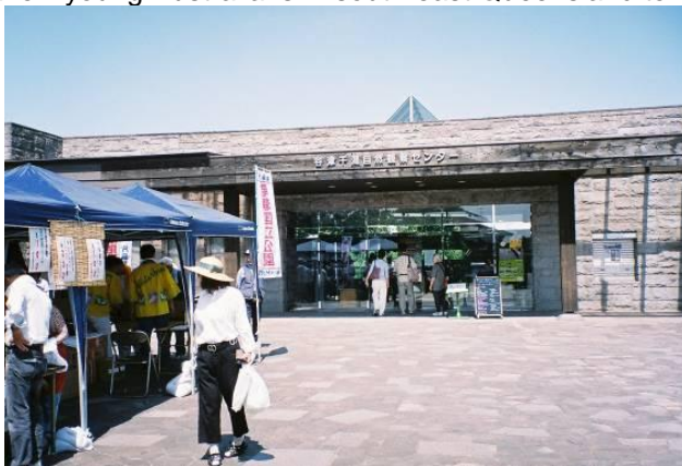
Entrance to YH Wetland Centre
